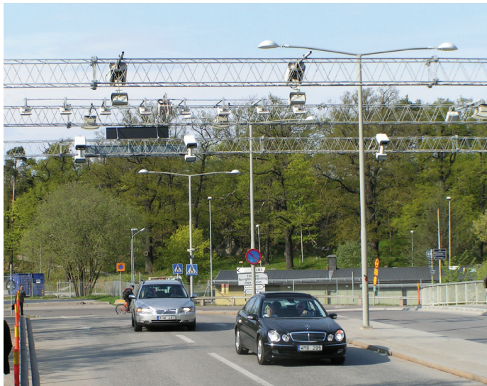
Cars arrive at an automated license plate scanning location while entering the city center
