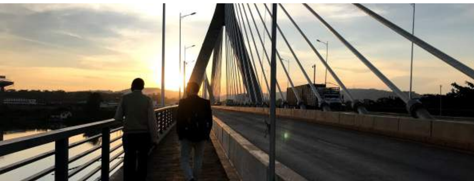
The New Jinja Bridge, the first cable-stayed bridge with pedestrian walkway and dual highway in Uganda, commissioned in 2018 restricts boda motorcycles from using it (Photo credit: Beatrice Ch'ng)
